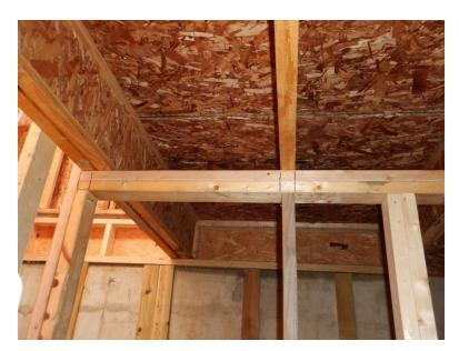
After plumbing the studs, toe nail them into the plates. Use Galvanized (SILVER) nails in to the PT bottom plate.
