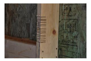
Place 2x4/2x6 wall cleats in cutouts and nail to each wall stud, with 2- 16d nails. Make cleats full length and attach to all studs.
