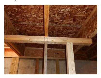
Cut the 2 x 4 studs to length and **position directly under TJI/floor joists and LVL**.
