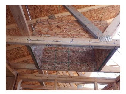
Nail the 31" pieces of OSB INSIDE the lines, with edges, flush with the bottom of the truss.
