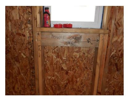
Towel racks 2 x 6 blocking 42" center of blocking from subfloor Mirror 2 x 6 blocking 69" center of blocking from subfloor Future medicine cabinet 2 x 6 39" center of blocking form subfloor
