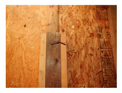
Place a 6' level on the bottom chord of at least 2 truss's, at the PEAK. Mark the 2 x 4 where the level touches it. Repeat the process on the other side of the PEAK.
