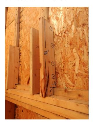
Place 2-  $2 \times 6$  at the peak of the cathedral truss, where the nailers will meet. Also, cut a piece of  $2 \times 4$ -- 12" long and nail between the  $2 \times 6$  's.
